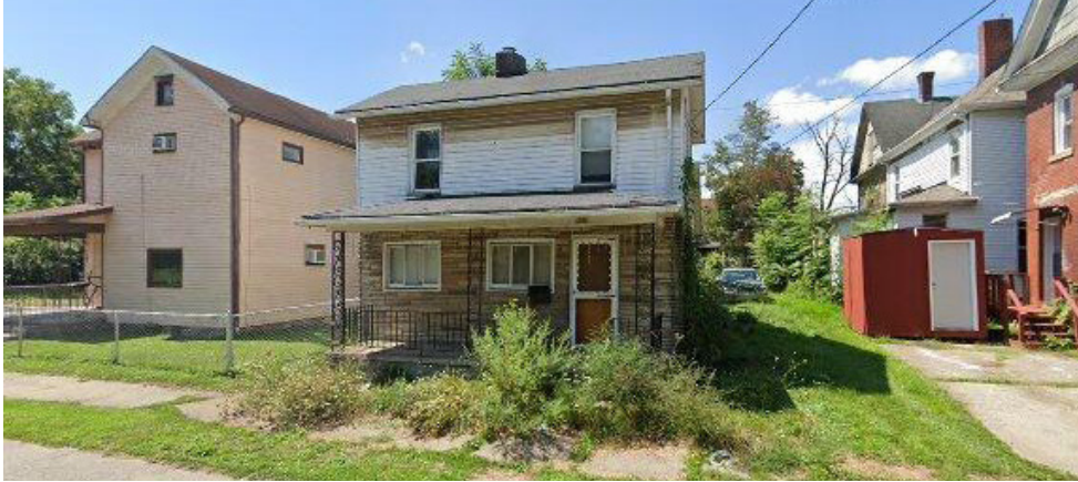
Figure 4. House (on the right) located at 506 Spruce Street New Castle, PA before retrofit, ( https://www.zillow.com/homedetails/506-Spruce-St-New-Castle-PA-16101/86510118_zpid/ ).
