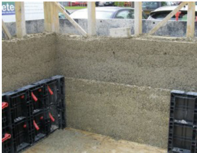
Figure 1. Example cast in place hempcrete wall confining studs (Left, Courtesy of American Lime Technology http://www.americanlimetechnology.com/tradical-hemcrete/ , and Right, Flahiff 2009: https://inhabitat.com/hemcrete-carbon-negative-hemp-walls-7x-stronger-than-concrete/ ).
