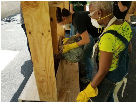
Figure 10. Mixing hemp hurd, lime and water to make hempcrete for cast in place demonstration by Americhanvre Inc.
