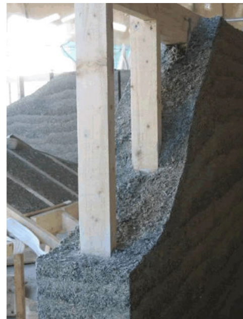
Figure 1. Example cast in place hempcrete wall confining studs (Left, Courtesy of American Lime Technology http://www.americanlimetechnology.com/tradical-hemcrete/ , and Right, Flahiff 2009: https://inhabitat.com/hemcrete-carbon-negative-hemp-walls-7x-stronger-than-concrete/ ).
