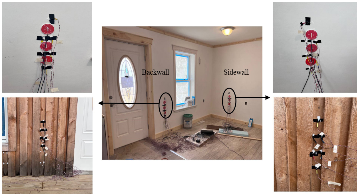
Figure 24. Overall connection setup in the house on two walls.
