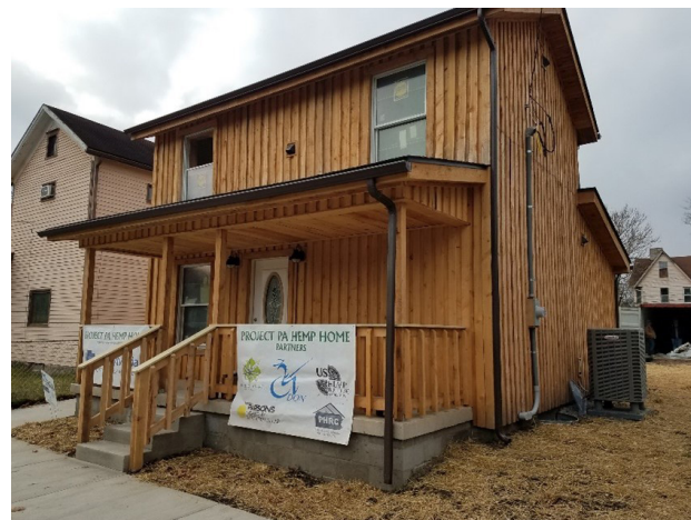
Figure 5. House after retrofit.
