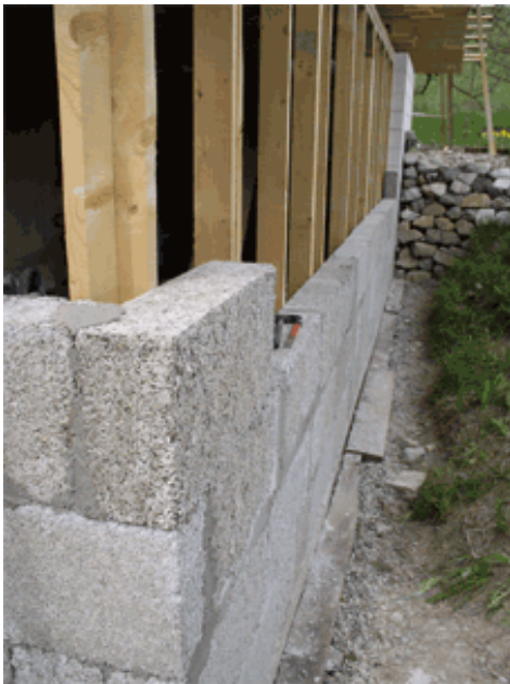
Figure 3. Typical example precast Hempcrete Block Building Construction (Below Left, Courtesy of Wikipedia: https://en.wikipedia.org/wiki/Hempcrete ; Below Right, https://www.iso hemp.com/en/hemp-blocks-buildings-hempro-system ).
